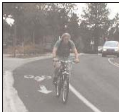
figure 2.3 Bike lane striping and pavement markings
