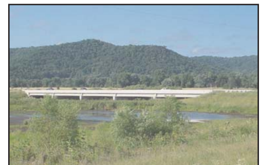
figure 4.8 Space for a pedestrian underpass has been provided in the design of the Mn 26 bridge at Miller's Crossing.
