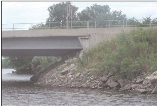
figure 3.7 Existing conditions at west end of West Channel Bridge.
