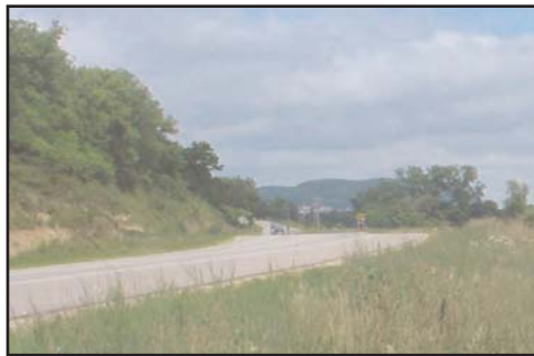
figure 4.6 Side slopes along Mn16 are not as steep as north of town along US 14/61.
