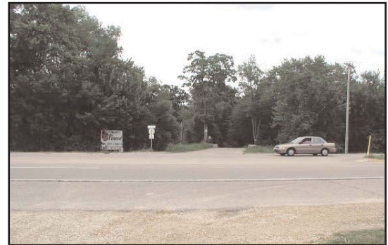
figure 3.6 Existing conditions at Old Monte Carlo Road crossing.
