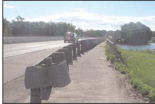
figure 3.8 Existing conditions on south side of West Channel Bridge
