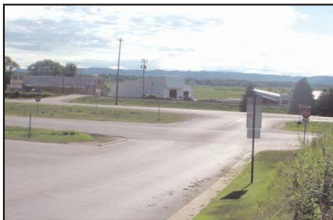
figure 4.4 Existing Mn16 crossing condition at S. 14th Street.
